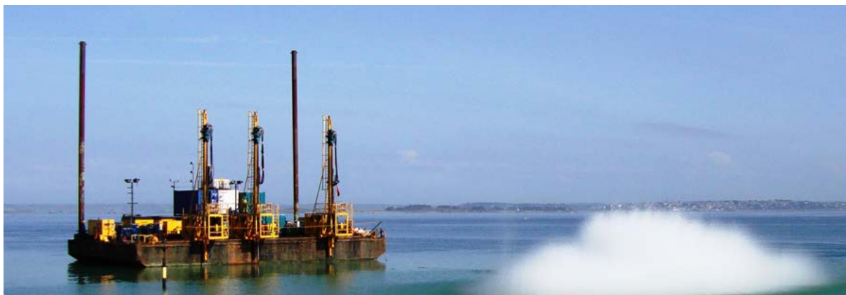
Figure 3-10. Controlled subsea rock blasting (Ramboll 2013).
