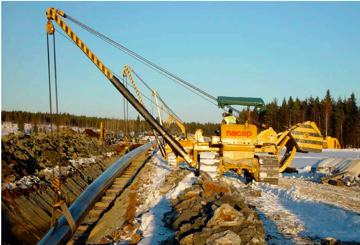
Figure 3-19. Example of a natural gas pipeline being laid (Gasum Oy).
