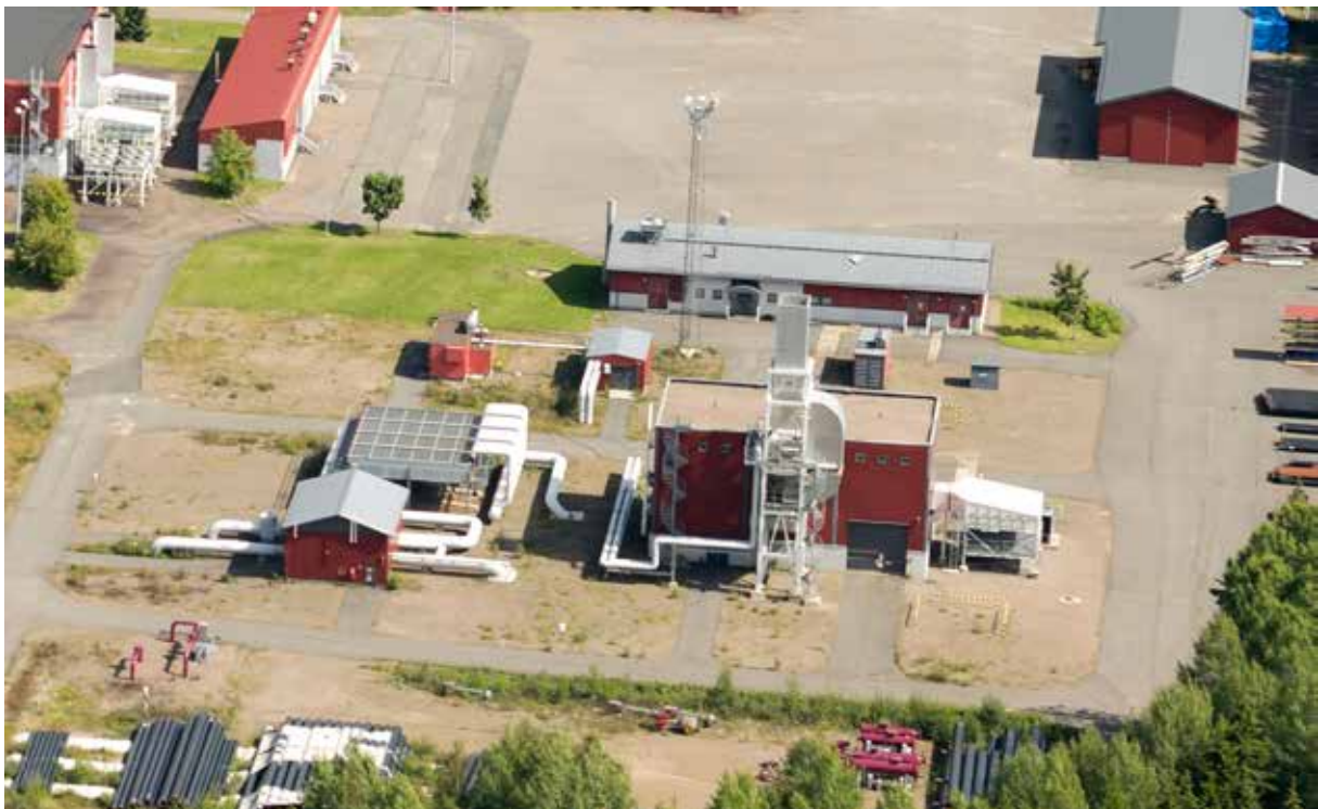
Figure 1.18. A 10MW gas turbine driven pipeline compressor station in Kouvola in Finland (Gasum Oy)
