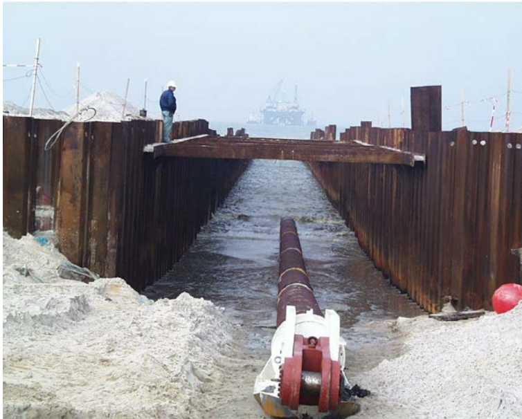
Figure 10-14 Pull-in head emerging from sea at shore pull
