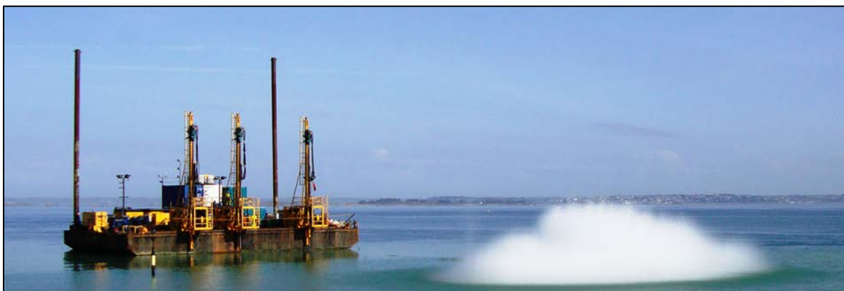
Figure 11-5 Controlled blasting of subsea rock
